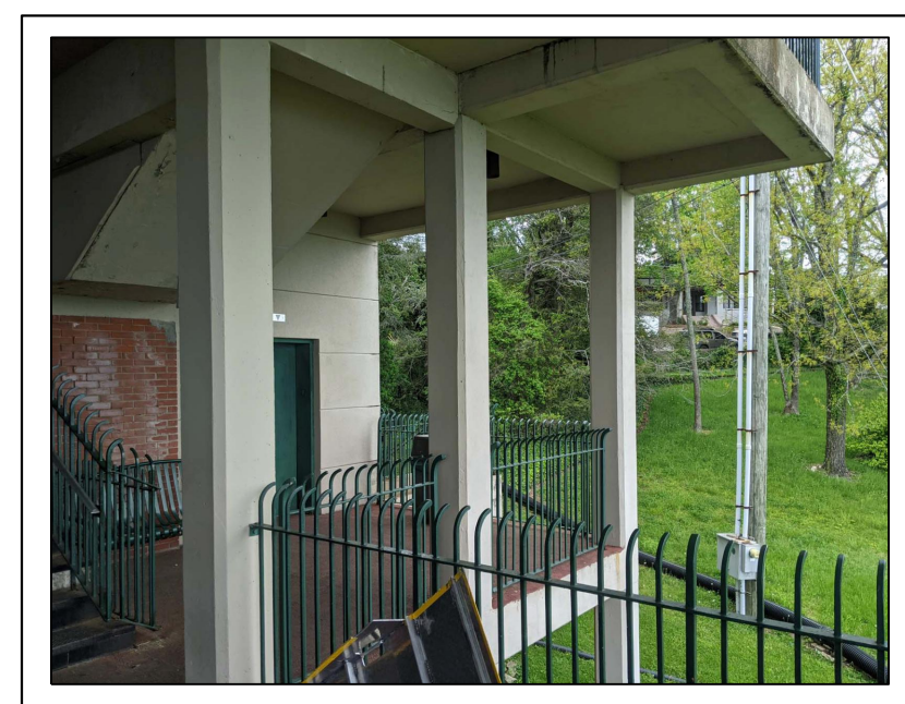
A STANDING ON LOADING PLATFORM NO. 1 AND LOOKING NORTHWEST TOWARD ELEVATOR
